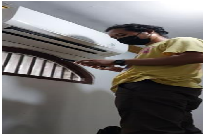
Gambar Survei sistem AC type Split Wall indoor
